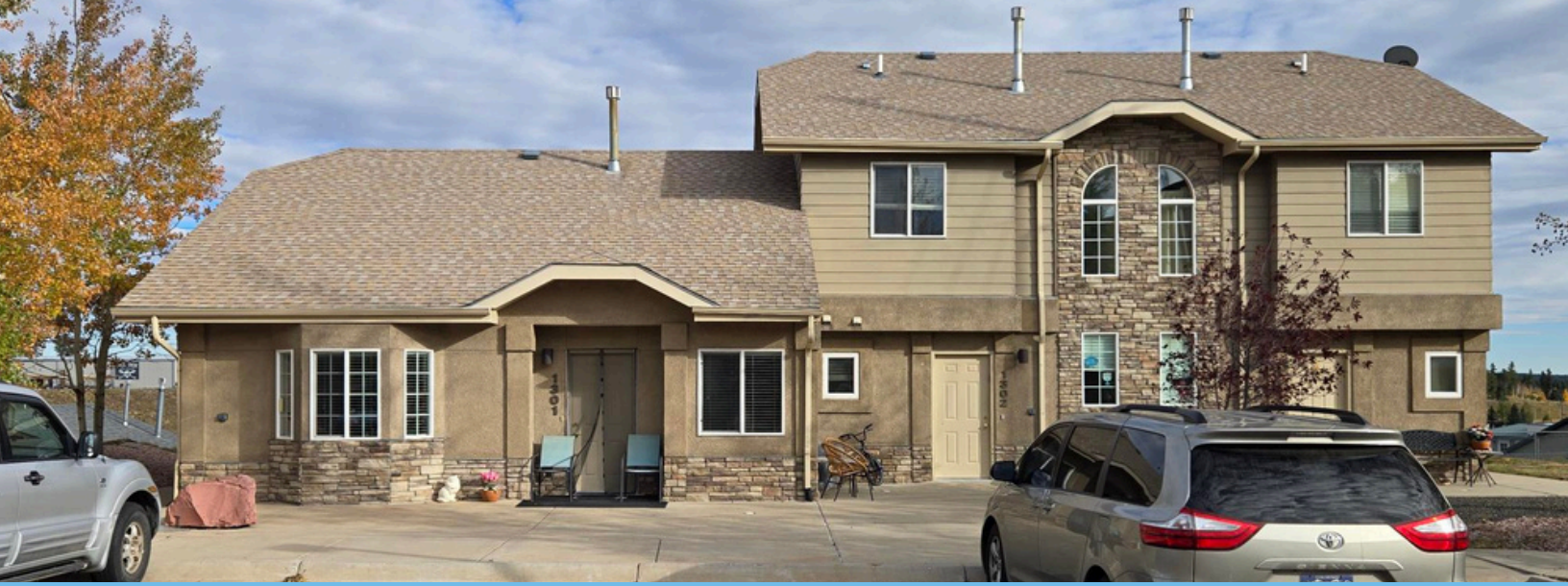
Hybrook Townhomes Photo courtesy of Greccio Housing
